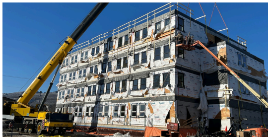
The Willows takes shape on the grounds of the old Howard House on 43 rd Avenue in Vernon
